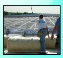
Once construction is complete, the mesh remains as a permanent part of the roof system, providing support for the insulation materials. The product's white color blends well with most fiberglass insulation facings, maintaining an attractive and nearly invisible appearance.
