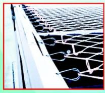
Naturally, the Green-Web system cannot protect against injuries from falls onto structural members. In addition, tie-off systems are still required for workers near the perimeter of the building and during the mesh installation process.
